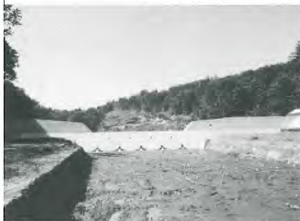
蓬田川治山ダム (長さ75m・高さ5m・体積1,046m 3 )
